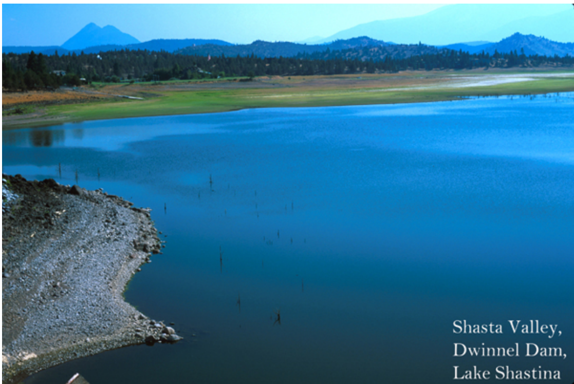
Figure 37. Dwinell Reservoir looking southeast off the dam with water levels at less than full pool in 2002. Long retention time and exposure to sunlight trigger algae blooms and nutrient pollution. Water releases from this reservoir are restricted to avoid adding to water pollution downstream. It has blocked downstream flow since 1928 in violation of CDFG 5937. Photo from KRIS V 3.0 by Michael Hentz.
